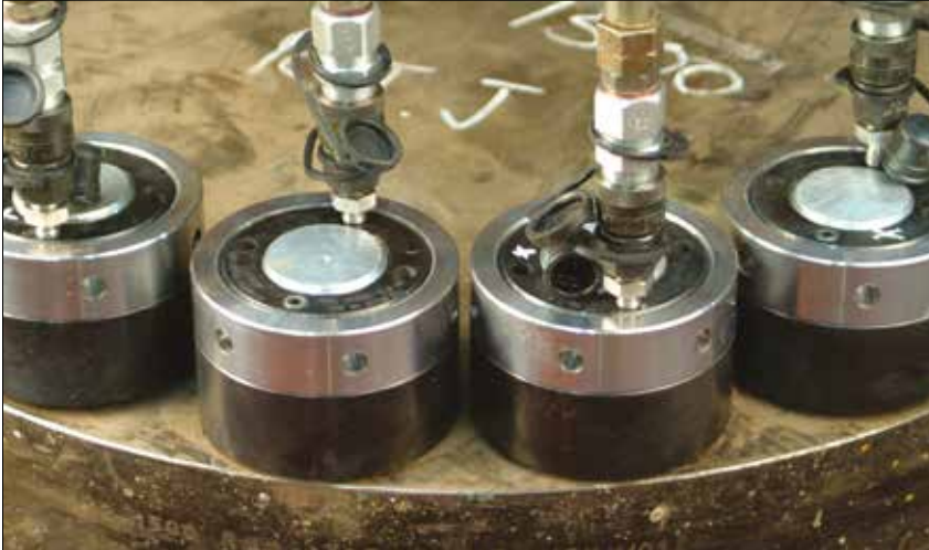
▲ Tensioning with hydraulic nuts.
