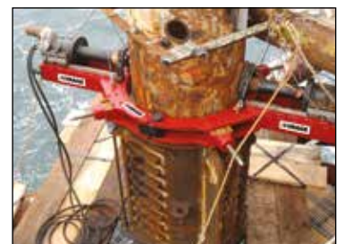
▼ DDU1636 casing pin drilling.
