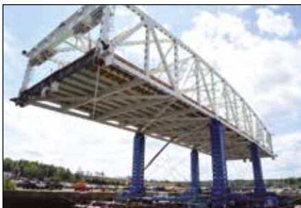
Incremental bridge lifting
