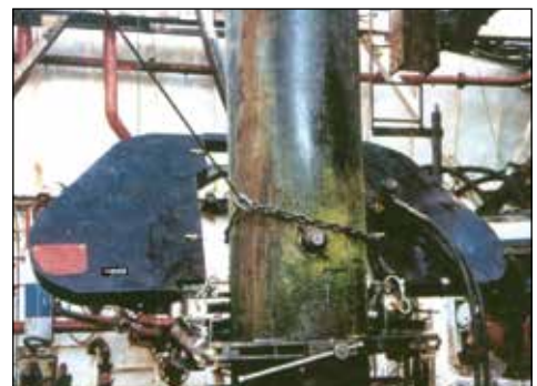
▼ Decommissioning job with band saw.
