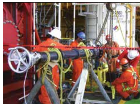
▼ CHT2000 hot tapping offshore application.
